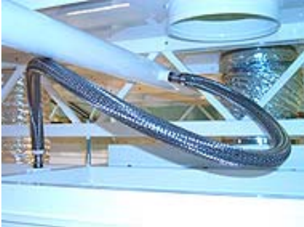
Typical flexible drop system used in Clean room application.
